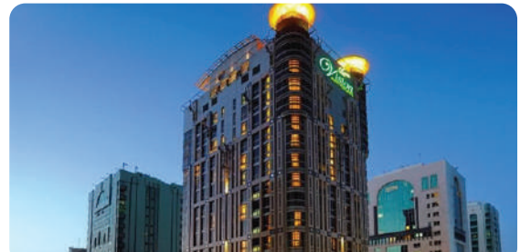
Digital HD TV System SMATV System IF CCTV System
