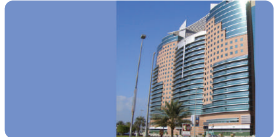
SMATV System CCTV System
